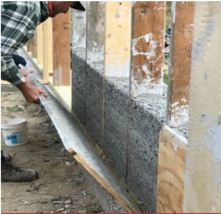
Roman Vyskocil and participants pouring, mixing, and revealing final hemperete wall.
