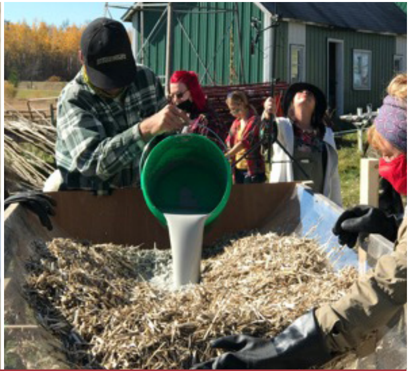
Roman Vyskocil and participants pouring, mixing, and revealing final hemperete wall.
